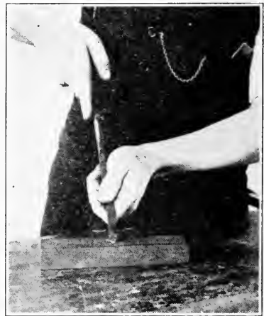
FIG. 53. PUTTING BURR ON SCRAPING CHISEL.
